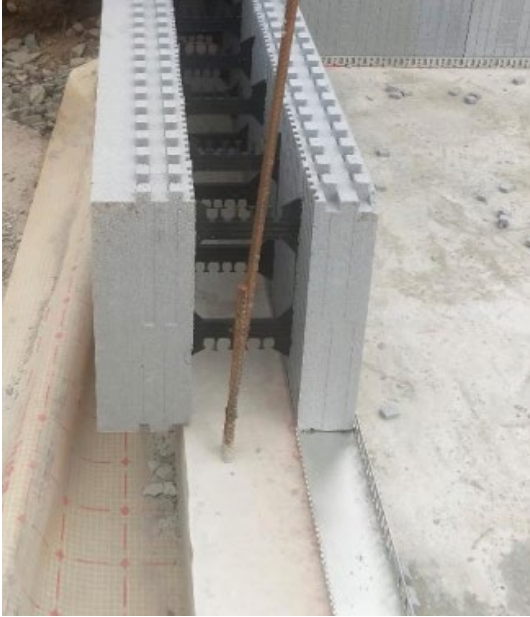
Figure 2: Castleforms ICF Therm Wall and Starter Track
