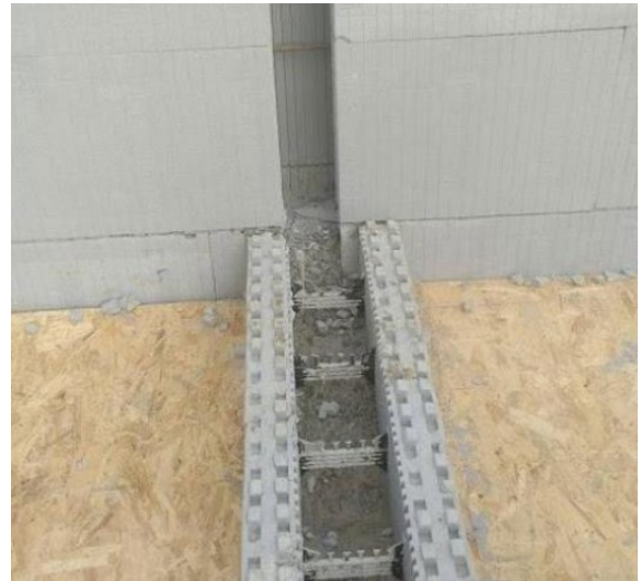
Figure 1: Construction of Compartment Wall
