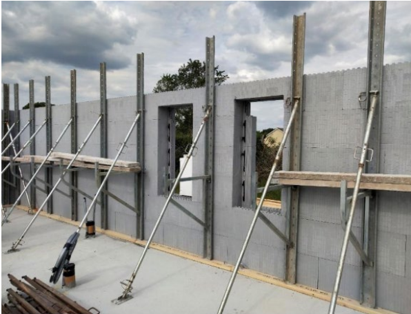
Figure 3: Bracing System for Castleforms ICF Therm Walls
